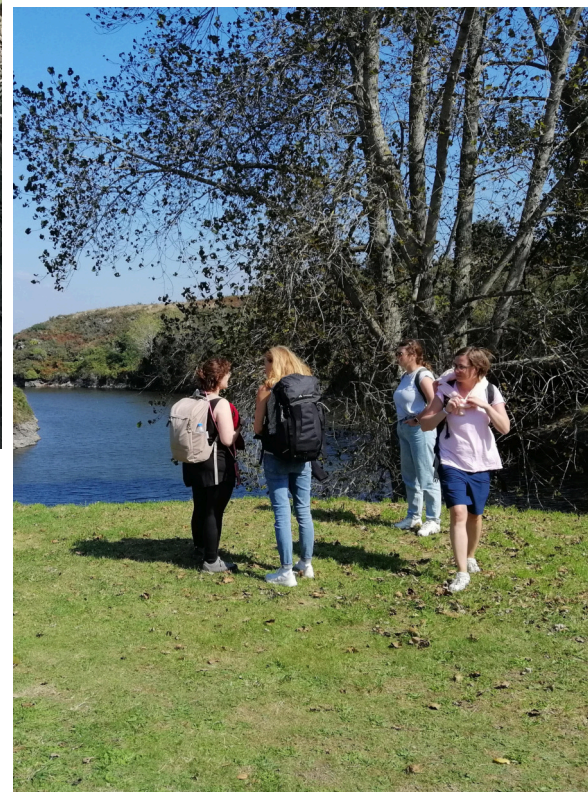
A stop at the dam to talk about water management on an island
